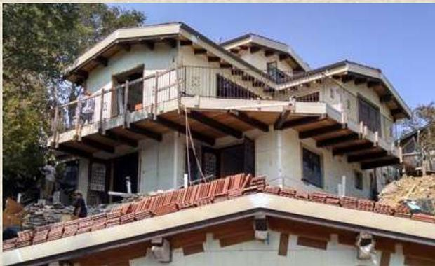
The **Shade/Nabben Residence** is concrete from the foundation to the roof ridge other than use of decorative wood for architectural appearance and a few steel stud wall partitions. The Integraspec building system is based on polystyrene foam concrete forms that when filled with reinforcement and concrete create a concrete wall insulated on both sides with 2.5" of high density foam.
